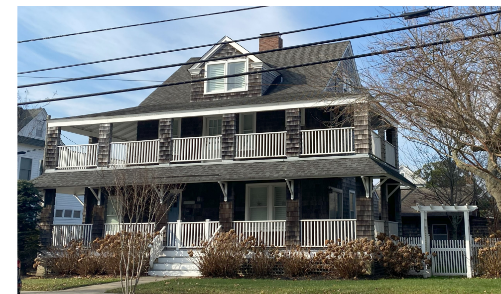
Examples of typical Bay Head houses; simple shingle-style residences, with two story porches facing east and south to benefit from the prevailing winds, to shade the interior spaces, and to provide a social space to the public street.
