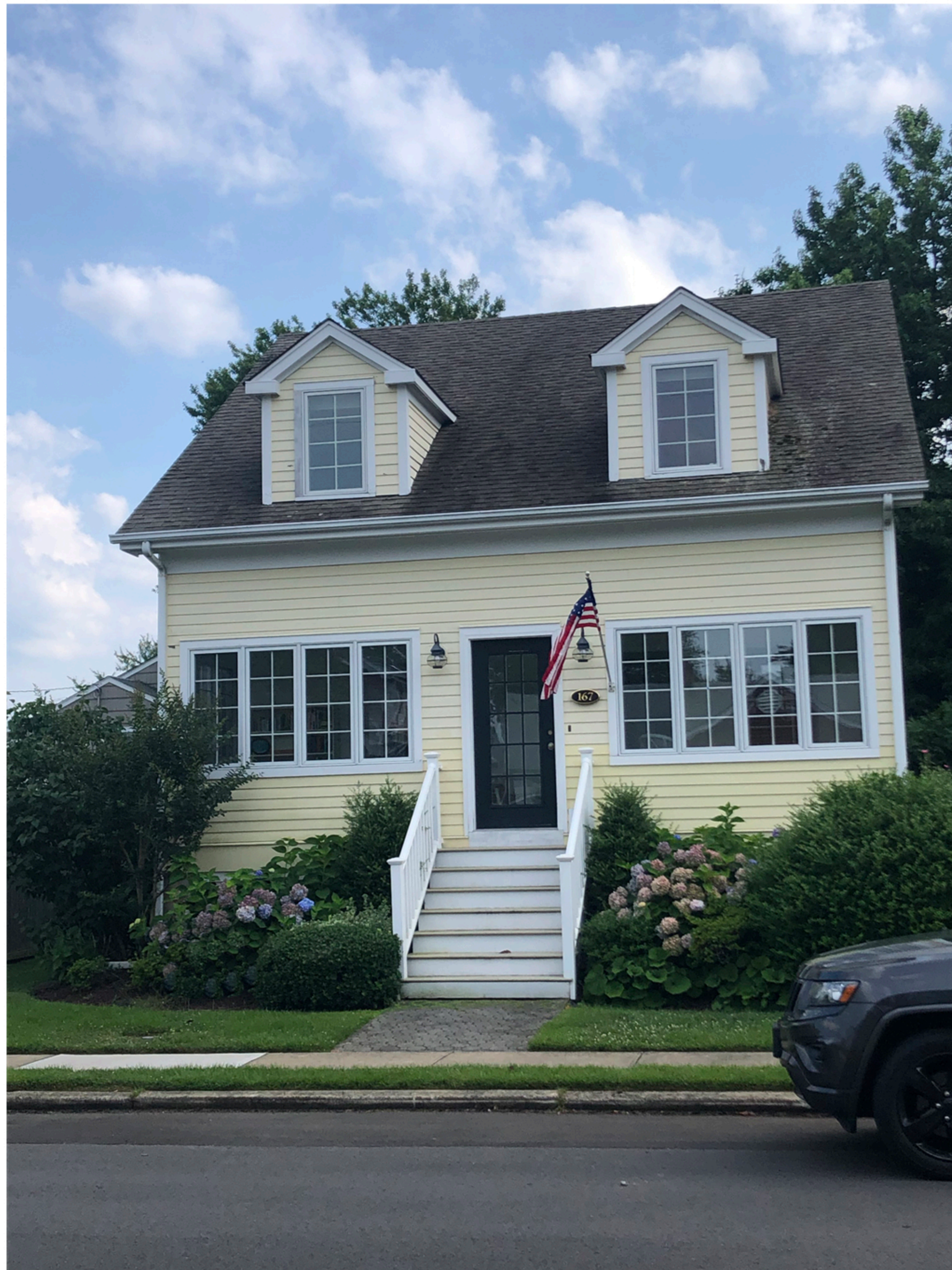
PHOTO OF EXISTING
