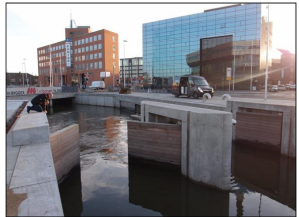
Image of Typical Tidal Flood Control Gate Considered for Scow Ditch, Bay Head.
